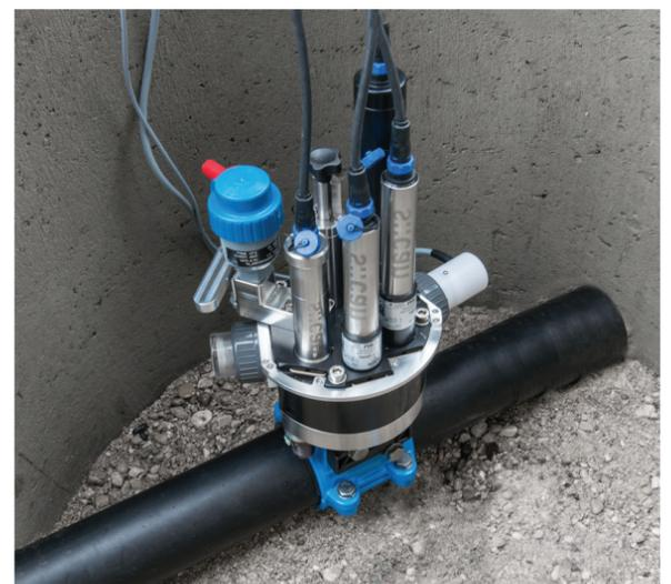
Figure 8: The pipe::scan is a sensor system for monitoring drinking water quality in pipes under pressure.
