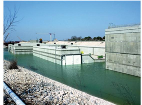
Caissons made of reinforced concrete form the foundation of the flood protection system: KELLER AG für Druckmesstechnik
