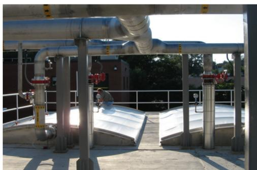
(GTI), the cover collects biogas and minimises heat loss. It also provides odor control and better corrosion resistance compared to concrete or steel. GTI has had success with similar covers at other food processing facilities.
