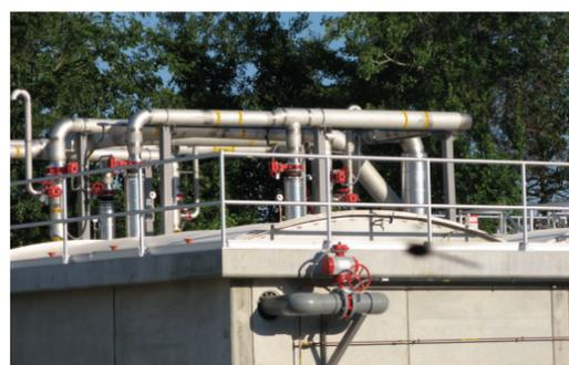
The very clean effluent from the AnMBR now goes into the old SBR, which has been repurposed for use as a sulfide oxidation and nitrification tank. Ken's purposely adds and maintains biological solids in the tank as a suitable biomass population for the treatment process. Now that solids loading to the SBR from the anaerobic process has been eliminated, the SBR can be easily used to oxidise sulfide and ammonia.
