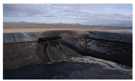
Fig. 1 Liquid effluent is pumped from finishing barns to a one million gallon influent basin.
