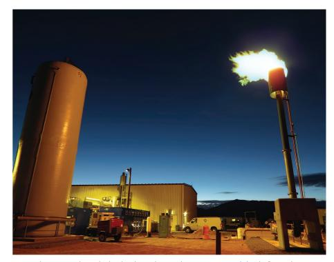
Fig.5. Methane gas is and passed either directly into the secondary gas compression skid or the flare stack.
