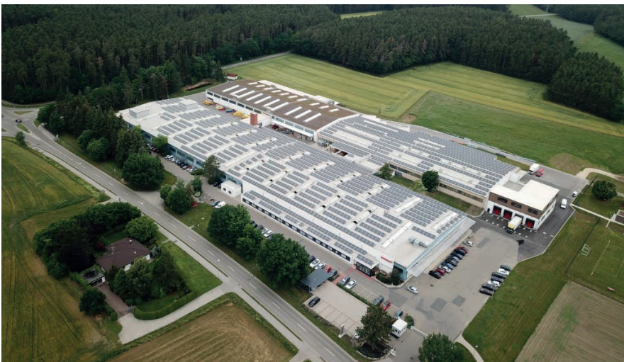
Memmert GmbH + Co. KG Production site in Buechenbach, Germany
